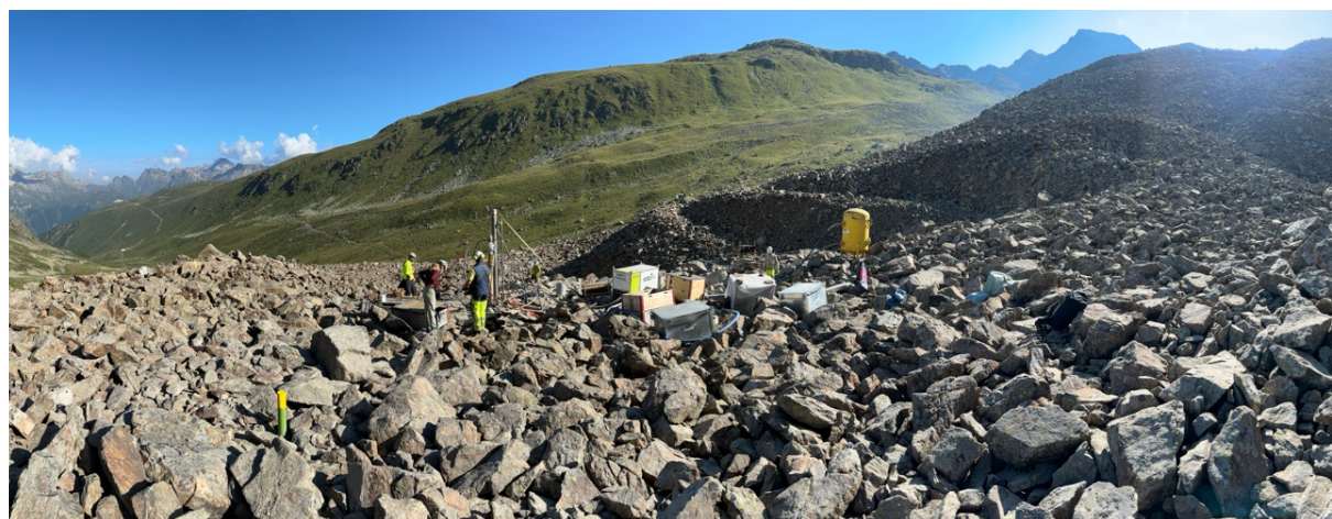
Figure 3.6. Drilling of a new borehole for permafrost temperature measurements on rock glacier Muragl in the Upper Engadine in August 2024. Photo: J. Noetzli.
